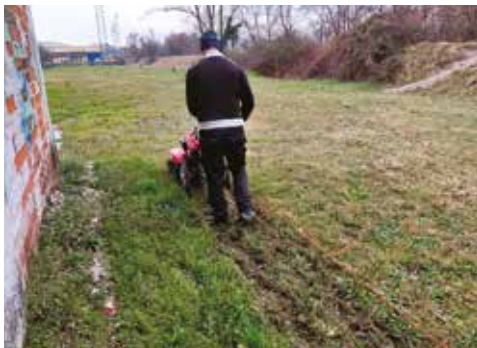
1. Surface preparation of the soil using a rotary tiller
