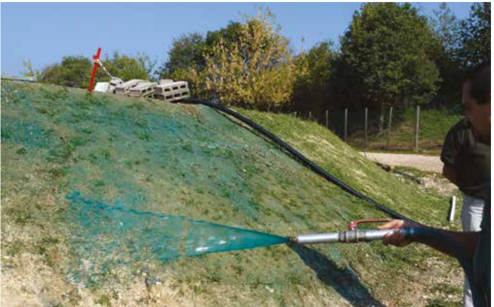
Hydroseeding of a mixture of native seeds on a small embankment. The green dye helps to better visualize the already seeded portion
