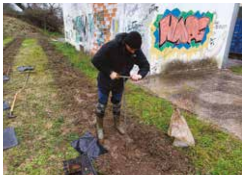
2. Excavation of the hole using manual mechanical equipment or a motorized auger
