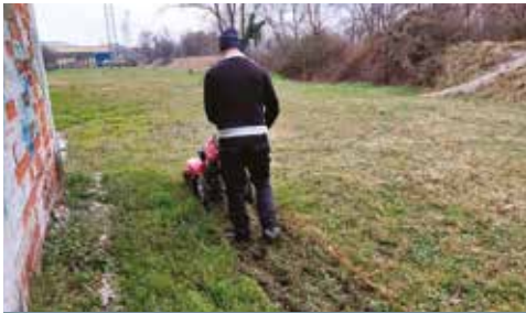
1. Surface preparation of the soil using a rotary tiller
