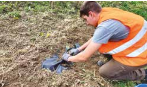
5. Manual filling of the planting holes and soil compaction
